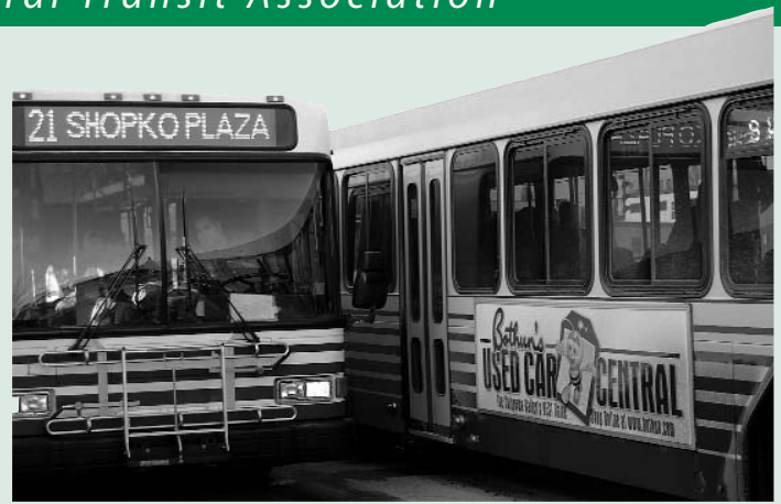
SQUEEZING BY – One of Eau Claire Transit's university route buses cannot pull all the way into the bus lane at the outdated Transfer Center. Because of the close quarters, one bus is forced to load/unload passengers mid-lane. A "temporary" structure built in 1985, the Transfer Center is literally falling apart, has no public restrooms and inadequate heating. The city planned to replace the Center in 2004, but the project has been repeatedly delayed by the lack of federal funding.
